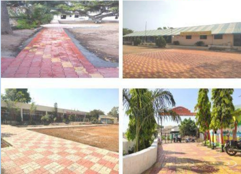
Laying of paving blocks
