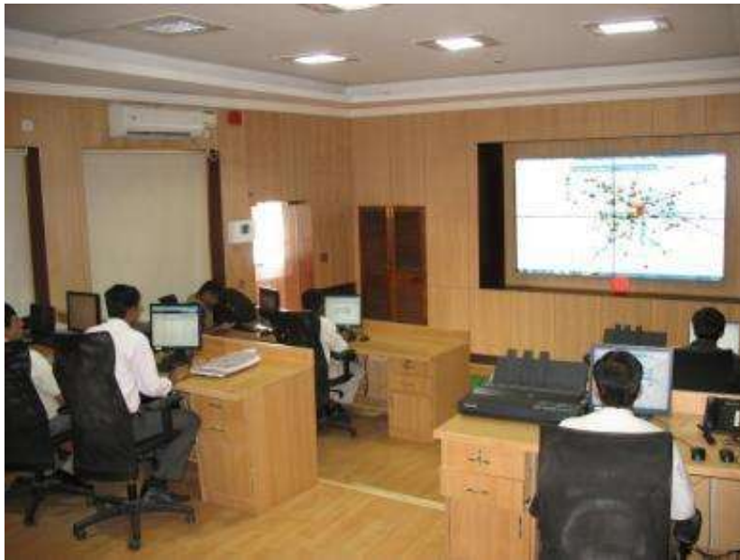
(ITS Control Room in Mysore City)
